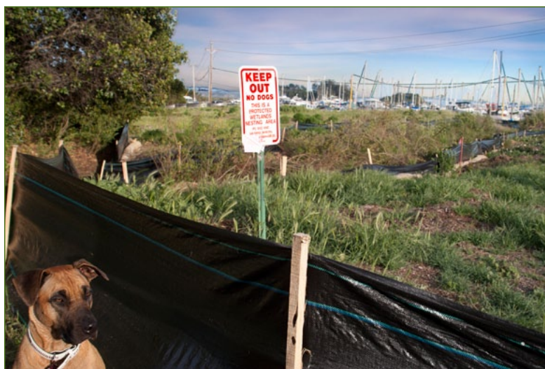
Construction-related mitigation measures at Loch Lomond Marina include the installation of temporary silt fencing to protect the wetland nesting area.
